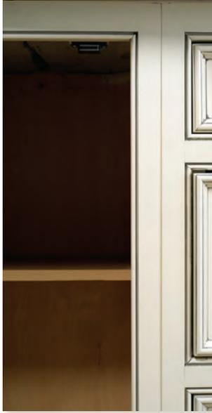
*When an inset door style is used, cabinet face frames can be beaded as shown in the photo to the left.*
